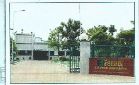
Oil seals Plant, Sriperumbudur - Tamilnadu
