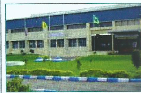
Engineering Product Plant, Pashamailaram - Telangana State
